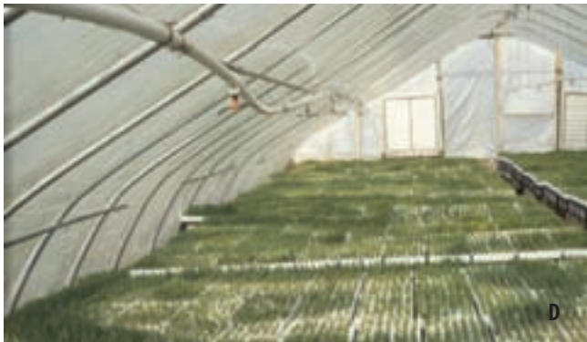
Figure 10.17 —(A) Because sprinklers produce a circular irrigation pattern, (B) proper spacing is critical to produce enough overlap. (C) The water pressure of irrigation systems should also be checked annually to make sure that nozzles are operating efficiently (D) before irrigation problems become apparent. Photos by Thomas D. Landis, illustration by Jim Marin.
