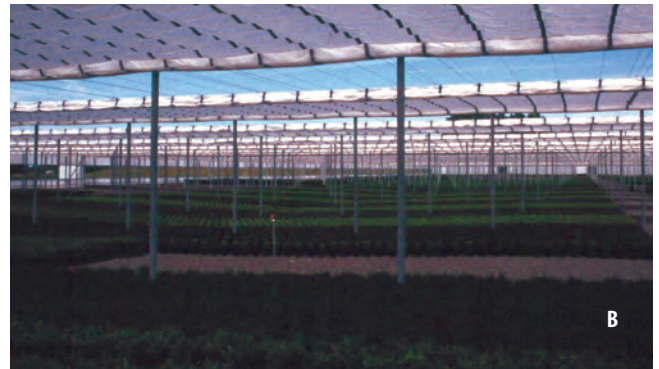
Figure 13.10 —(A) Fully enclosed greenhouses can be used for overwintering sensitive species but snow removal is necessary in cold climates to prevent damage. (B) Retractable-roof greenhouses are better for overwinter storage because they can be opened to allow snow to cover plants. Photos by Thomas D. Landis.
