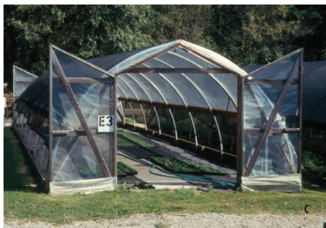
Figure 13.8 —(A) Polyhuts are low structures covered with white plastic or (B) a “sandwich” of poly film and Microfoam™. (C) The ends can be opened for ventilation during warm and sunny winter weather. Photo by Thomas D. Landis, illustration by Jim Marin.
