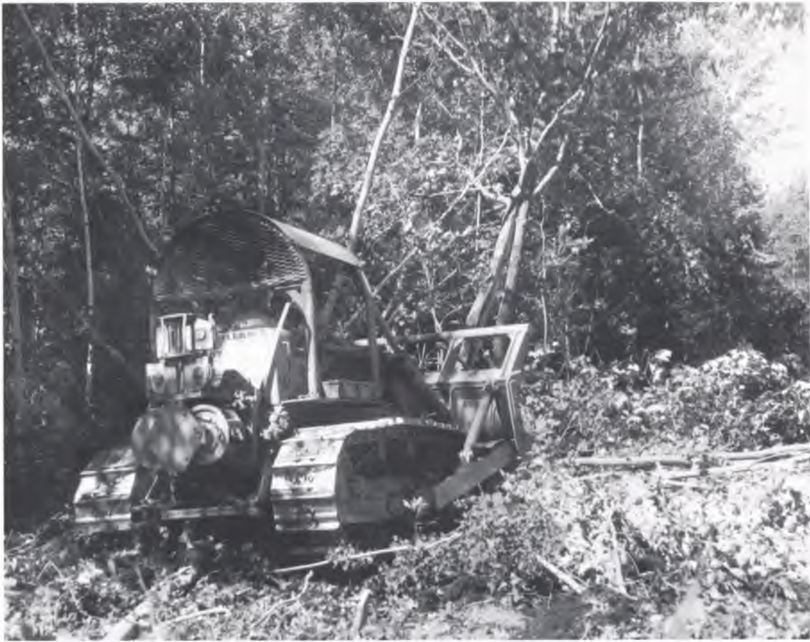
Fig. 1.--Diesel tractor with K/G blade clearing aspen stand to prepare site for planting spruce, Itasca County, Minn. (Photo supplied by M. J. Latimer.)
