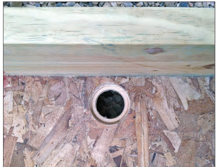
Figure 6. Drain assembly for subirrigation tank using a 1-in heavy duty polypropylene tank fitting with a 2.25-in hole size. (Photo by Tammy Parsons, 2015)
