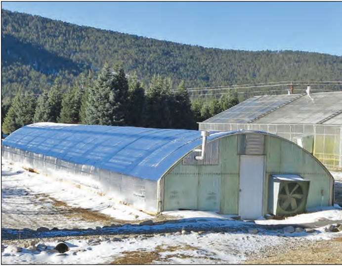
Figure 3. Modified cold frame using EcoFoil radiant barrier during winter at the John T. Harrington Forestry Research Center in Mora, NM. (Photo by Owen Burney, 2013)
