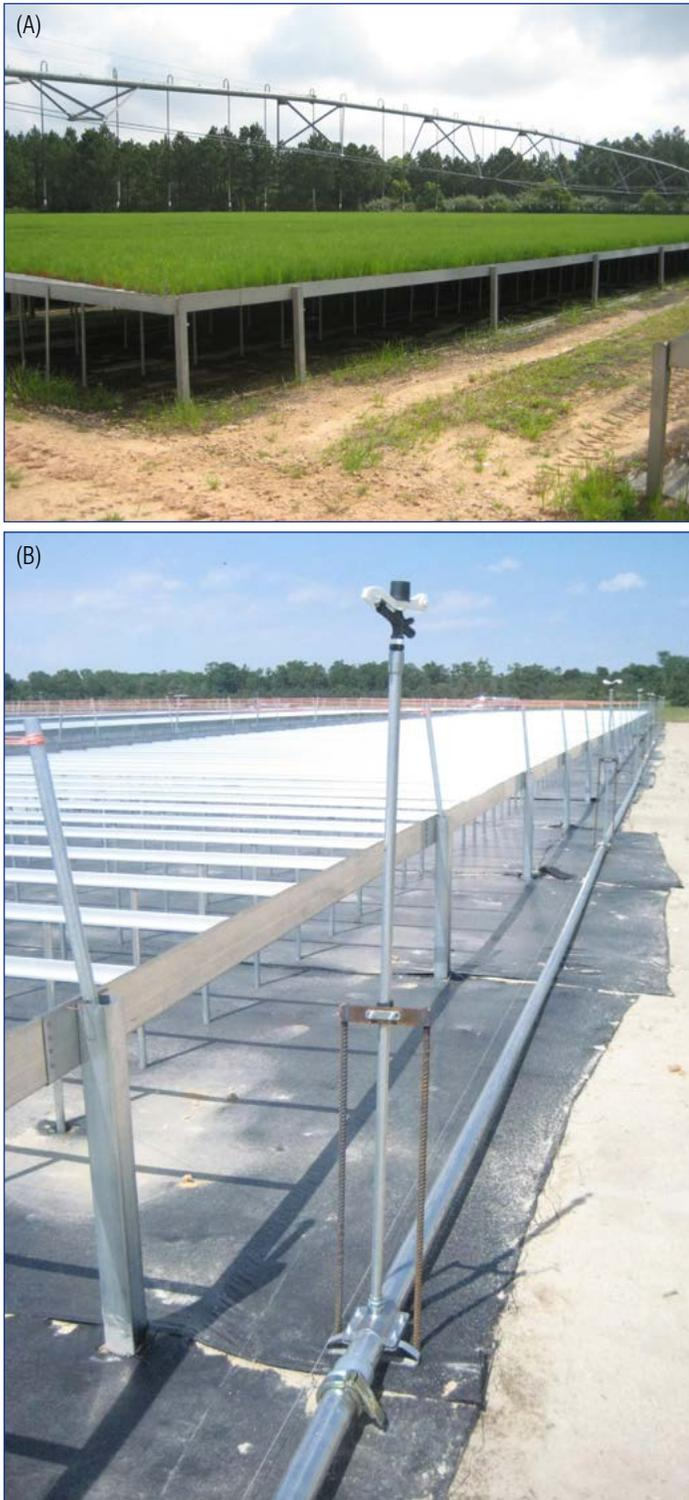
**Figure 4.** Irrigation systems used in southern container forest nurseries include (A) a center pivot irrigation system on benches and (B) a stationary impact head on a "T"-rail bench system. (Photos by Tom Starkey 2009 and 2010)
