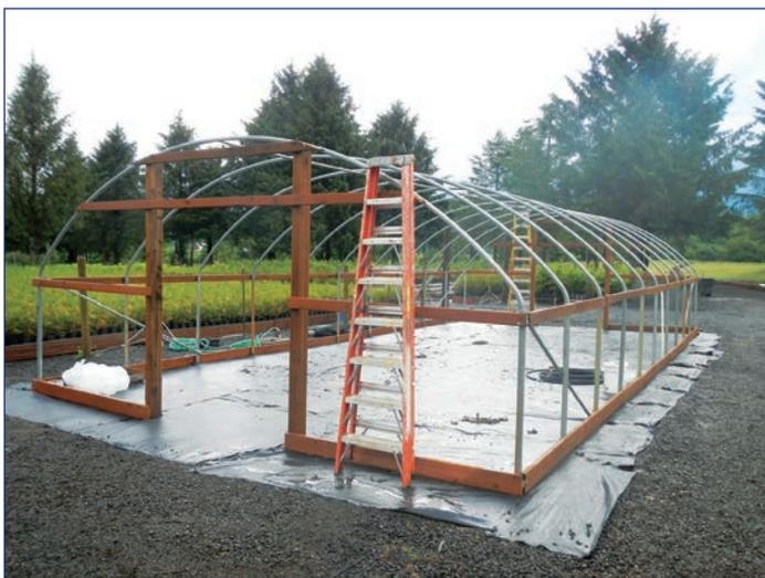
**Figure 13.** Shade house being constructed at the Oregon Youth Authority Camp Tillamook Work Study Center to use for direct sowing and outdoor natural stratification over the winter. The shade cloth protects seed from bird and rodent predation yet allows for ambient temperatures and rain. (Photo by Kurt Heckerth 2012)
