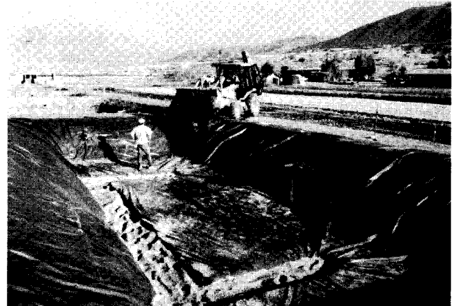
Figure 2—Smallest pond during construction, showing subsurface drain system and 30-mil plastic liner.
