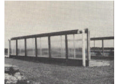
Figure 3. —Hotbed with sashes raised to storage position. Air intake and outlet pipes are located on the east and west ends of the bed, respectively.
