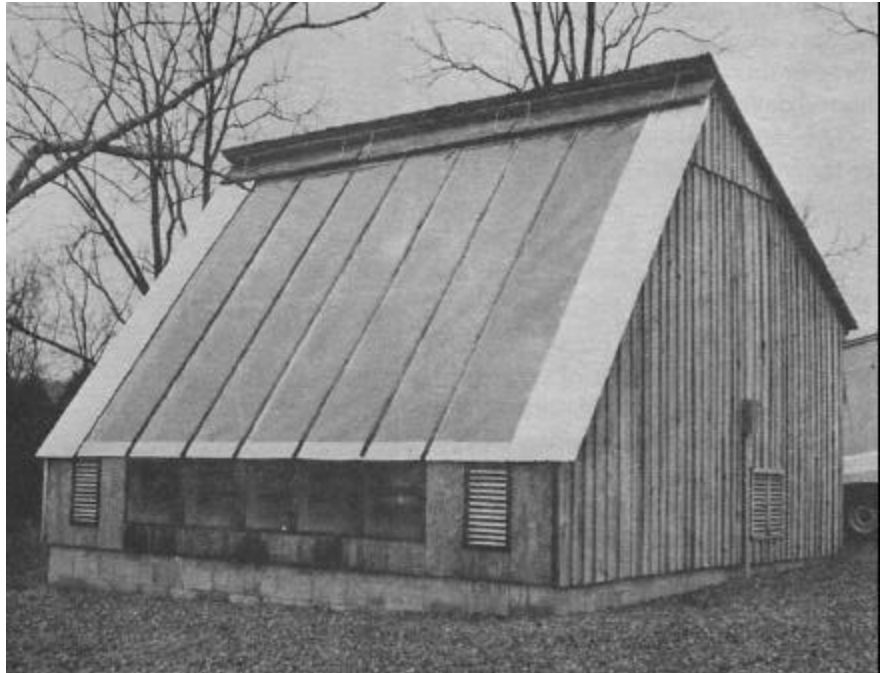
Figure 1. – Exterior view -south and east sides of solar-heated forest tree seed processing facility showing construction and collector details.
