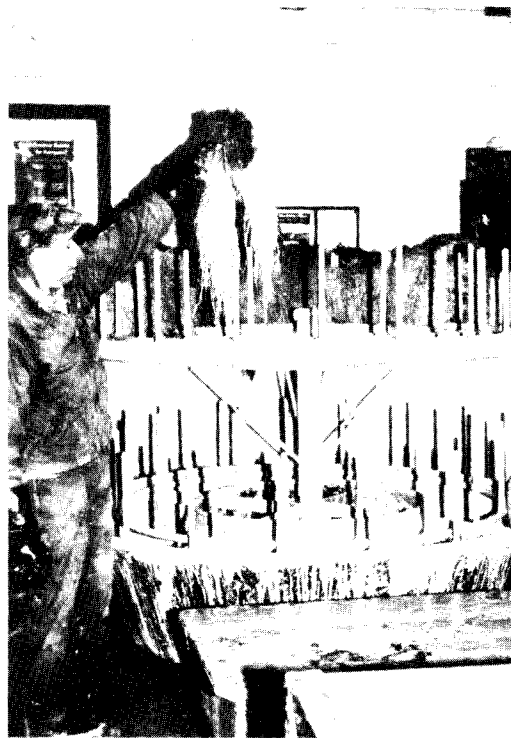
Figure 10-3. — Packing with clay slurry.
