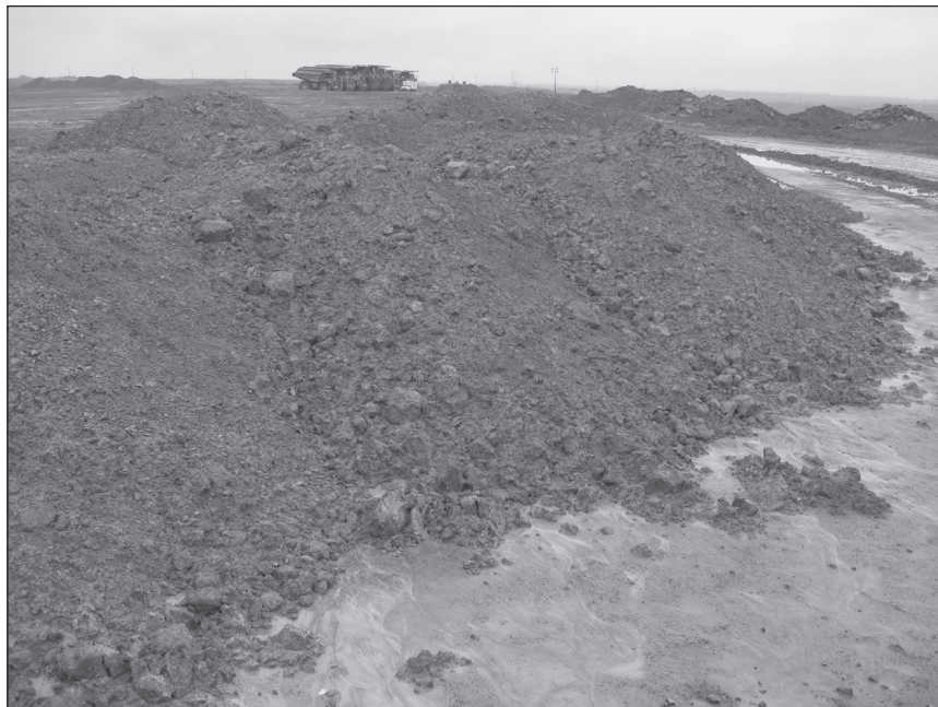
Figure 7. Replacement of soil after mining.
