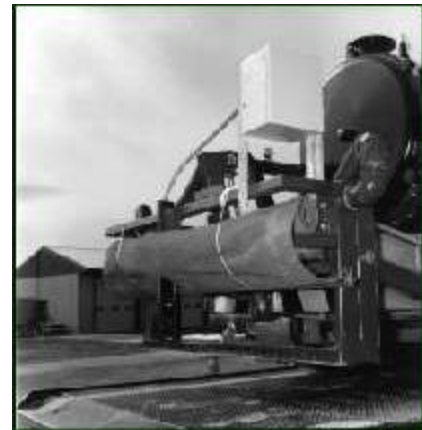
Figure 3. The initial steam injection system used an undercutter blade. Steam was vented from the back of the blade.
