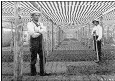
Figure 1. Horizontal overhead snow-fencing, "Pettis frames".
