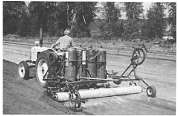
Figure 1 - Continuous tarp fumigation consists of glued, overlapping sheets of fumigation tarp which form a solid cover.
