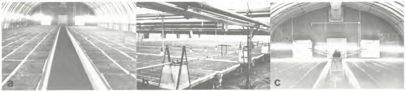
Figure 6. Some different lighting systems used for photoperiodic lighting: a) static incandescent; b) mobile incandescent; c) mobile VHO fluorescent.
