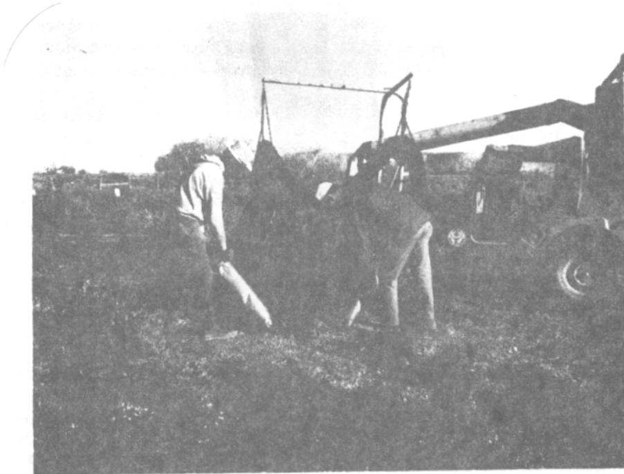
Fig. 2.--One model of vacuum seed harvester being used to pick fourwing saltbush fruits off the ground.
