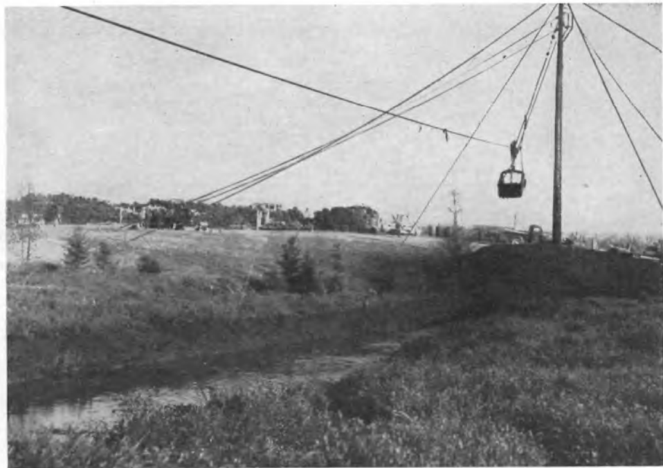
FIGURE 24.—A dragline set-up used in removing peat from spruce swamps. (Hugo Sauer Nursery, Rhinelander, Wis.)
