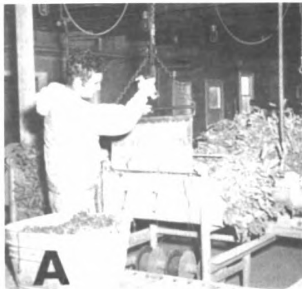
Figure 49.—Baling European alder seedlings at the Illinois Mason State Nursery: A, Belt-type baler operated by electric hoist; B, forming a veneer-mat bale.
