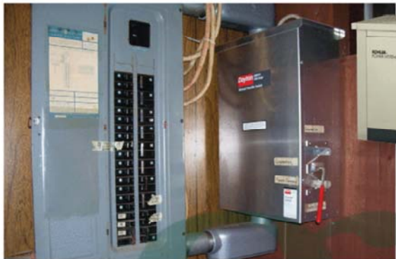
ABOVE: Generators are usually rated for continuous duty and load. Heavy-duty units will take considerable intermittent overload that helps in starting larger motors. LEFT: Except for a small standby generator that you can use to plug in a few lights or small motor, all units should be connected to the electrical distribution box by a transfer switch.
