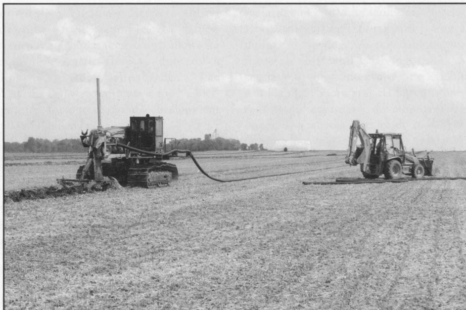
Corrugated HDPE pipe has a perforation pattern for subsurface drainage. Typically, four-inch diameter pipe is used, delivered in 3,000 foot-long coils and installed with a self-contained plow.
