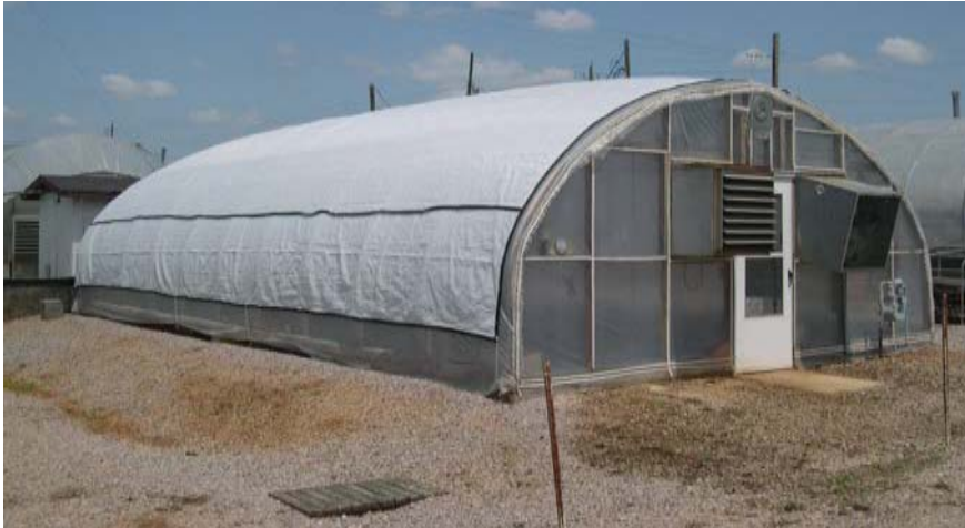
For externally-mounted shade cloth, a 60 percent reflective shade material was found to reduce the greenhouse heat gain by approximately 30 percent.
