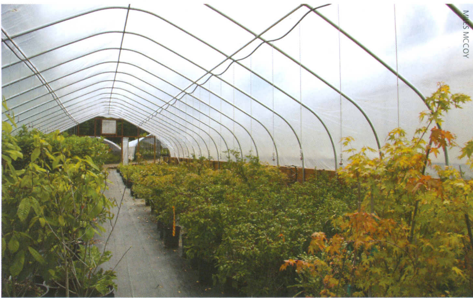
Polyethylene film (shown here) is the most common greenhouse covering in use today. Other common coverings include corrugated polycarbonate, and polycarbonate structured sheets (PCSS).
