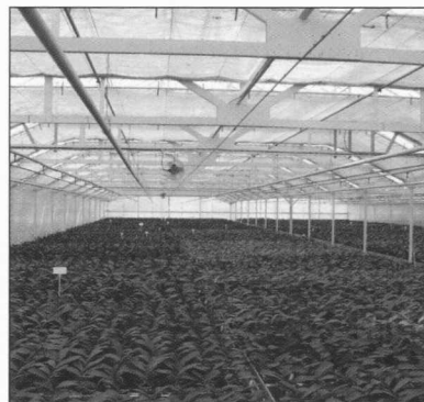
A curtain system installed in a "slope-slope" or "slope-flat-slope" profile allow the curtain to operate below the gutters but above truss-mounted or suspended equipment.
