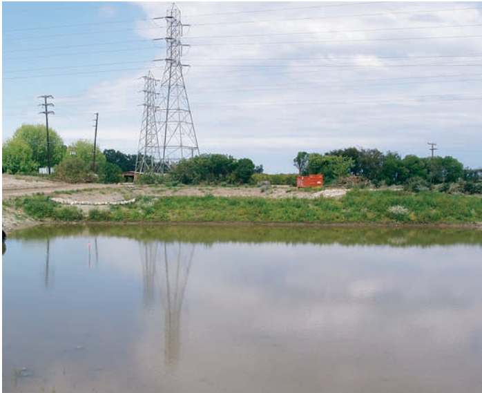
The unlined bottom of this detention basin allows captured runoff to percolate slowly into the ground. Soils and vegetation remove some contaminants from the water as it percolates or is taken up by plants.
