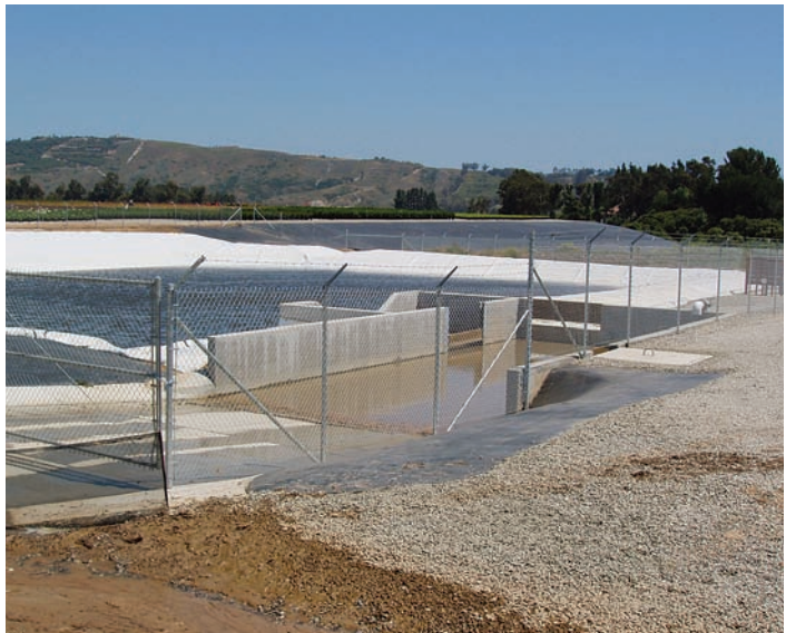
A retention basin allows runoff to be treated and recycled for use as irrigation water. Ventura County nurseries that recycle irrigation runoff significantly increased from 6% in 2004 to 14% in 2006.
