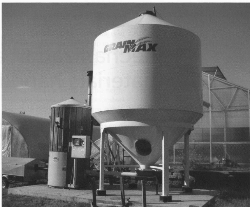
Commercial sized pellet boilers and bulk storage bins for pellets are an option for replacing traditional fuel such as propane.
