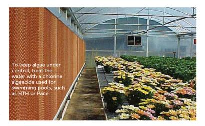
system to supply at least ½ gallon of water per minute per linear foot of pad system. The sump (tank) should be sized for a capacity of at least 34 gallon per square foot of pad area.
