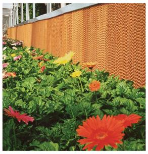
To get the optimum performance from an evaporative cooling pad system, make sure that all of the air entering through the greenhouse opening passes through the pads.
