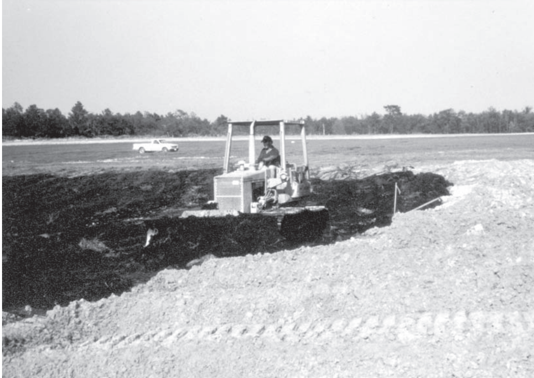
Figure 9.5. Bulldozer spreading topsoil at Hall's Branch restoration site.
