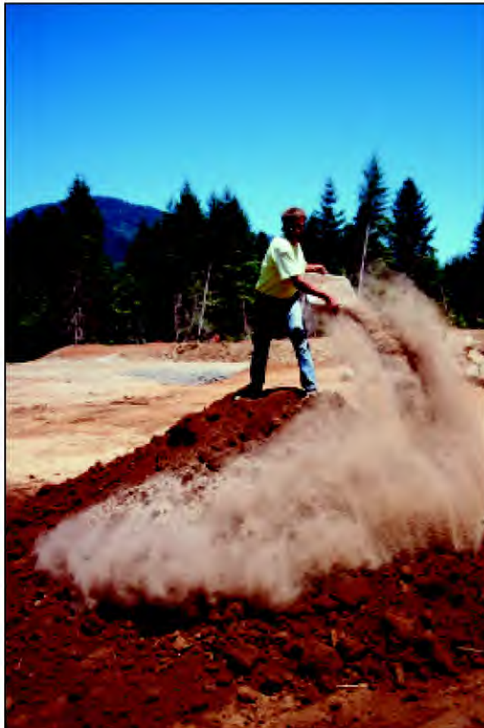
Topsoil was manufactured on site using loam from an alluvial deposit and mixing it three bucket loads of loam to one bucket of compost. Lime, slow release fertilizer, and mycorrhizae were added and then thoroughly mixed in.
