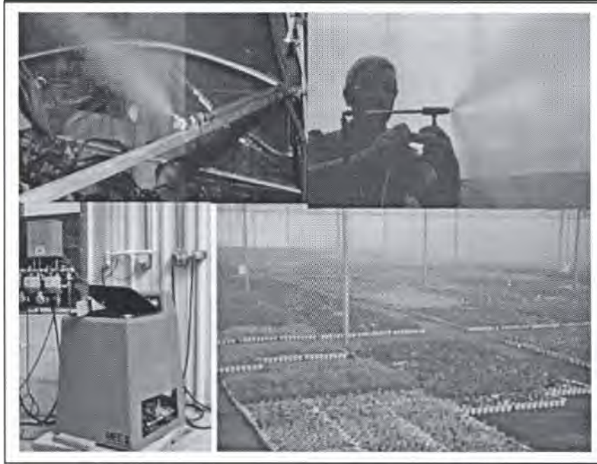
Figure 4. Fog systems form fine water droplets with an average size of 15 \mu\text{m} . Fog has a high surface: volume ratio, which helps water remain suspended in air as a vapor (gas) to maximize evaporation. Fog does not condense, avoids over-saturation of media and foliar leaching, which occurs with mist.
