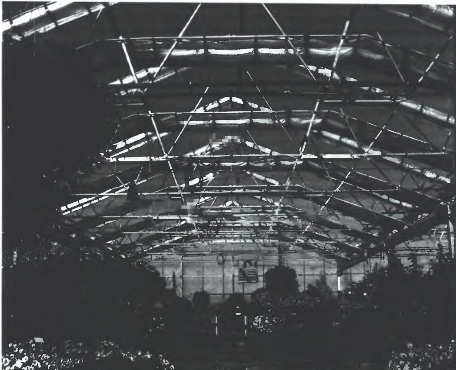
The A-Frame retractable-roof greenhouse manufactured by Cravo Equipment Ltd. offers maximum light and heat when the roof is retracted and maximum cooling when the roof and energy curtain are closed in opposite directions.
