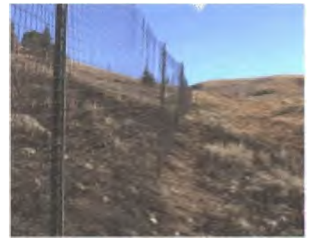
Figure 5. Plastic mesh fence, 7.5 ft tall (2.3 m), is supported by steel T-posts and high-tensile wire.
