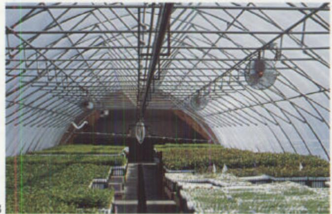
**Figure 6.4.7**—The importance of proper temperature is well illustrated by the shoot growth of these Colorado blue spruce seedlings—both too warm and too cool temperatures depress growth (A). Horizontal airflow fans (B) promote lateral air movement and help eliminate hot or cold spots with a greenhouse as well as supply carbon dioxide to the seedlings. (A, modified from Young and Hanover 1978).
