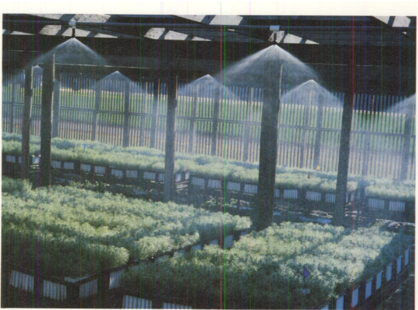
Figure 4.2.25 —Any irrigation system should be designed to provide overlap between individual sprinkler heads, particularly in outdoor growing areas where wind interference is likely.
