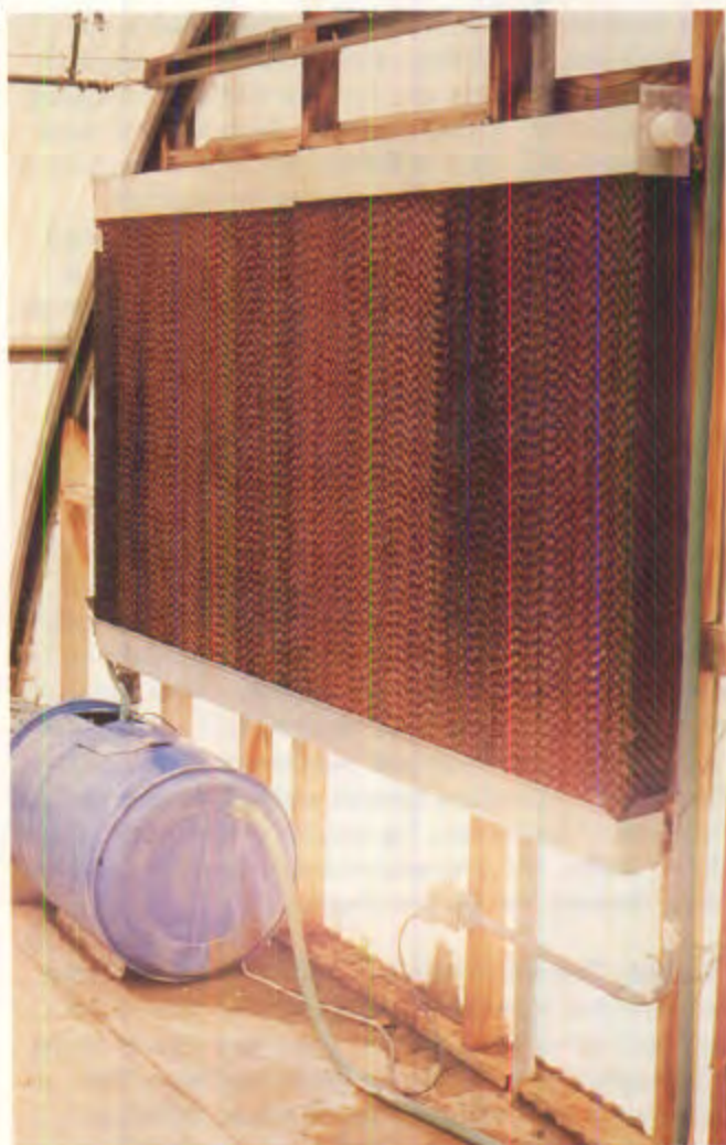
Figure 1.4.1 —Propagation environments can be cooled by reducing sunlight with shade cloth (A), increasing horizontal air circulation with fans (B), or with evaporative cooling by drawing air through a wet wall (C).
