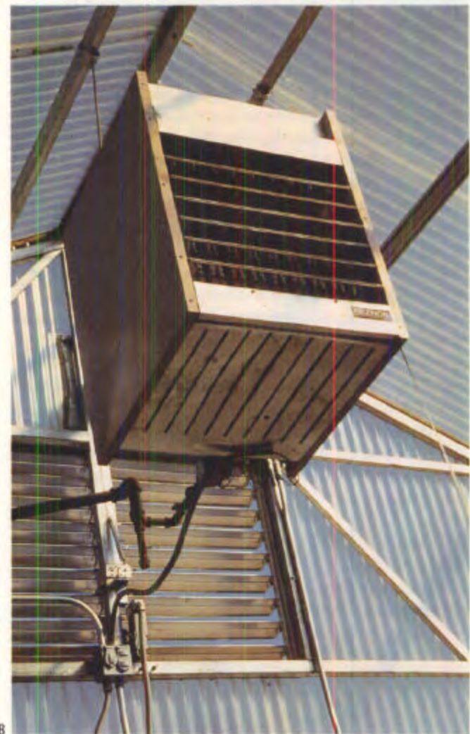
Figure 1.4.2— Propagation structures can be heated with a large central boiler, which distributes hot water or steam through pipes (A), or with unit heaters, which blow warm air directly into each propagation structure (B).
