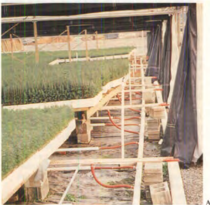
Figure 1.4.2— Propagation structures can be heated with a large central boiler, which distributes hot water or steam through pipes (A), or with unit heaters, which blow warm air directly into each propagation structure (B).
