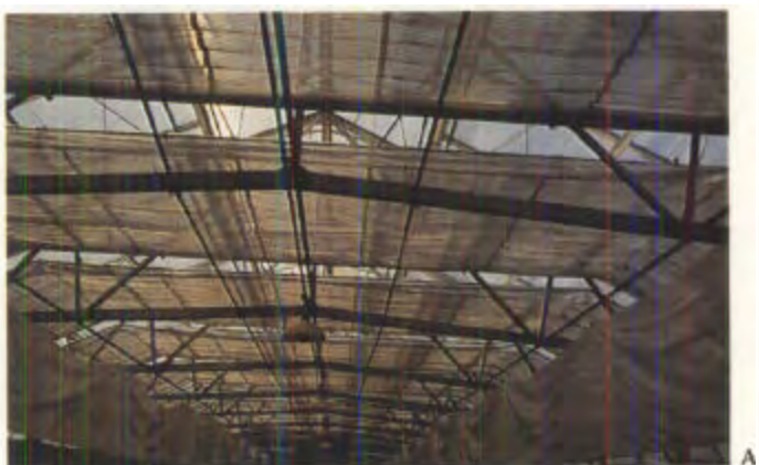
Figure 1.4.1 —Propagation environments can be cooled by reducing sunlight with shade cloth (A), increasing horizontal air circulation with fans (B), or with evaporative cooling by drawing air through a wet wall (C).
