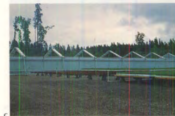
Figure 1.3.5 —Semiconrolled propagation structures are designed to allow easy and quick modification of the growing environment, from raising the sides (A) or adjusting the covering on the roof (B & C) (B & C, courtesy of Richard Vollebregt, Cravo Equipment Ltd.).
