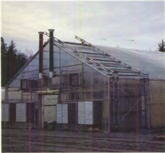
Figure 1.3.19 —Some nurseries use special scaffolds to make changing coverings easier and safer (A) and used plastic sheeting can now be recycled if it is rolled or baled (B & C) (B & C, from Bartok 1993.)
