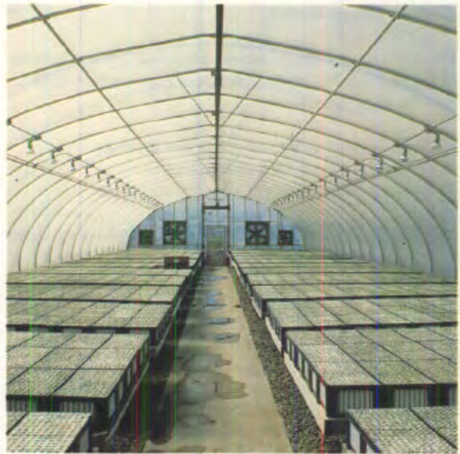
Figure 1.3.10 —Solid floors help keep the propagation environment clean and allow the use of handling equipment (A). Other structures feature traffic paths down the center aisle (B).
