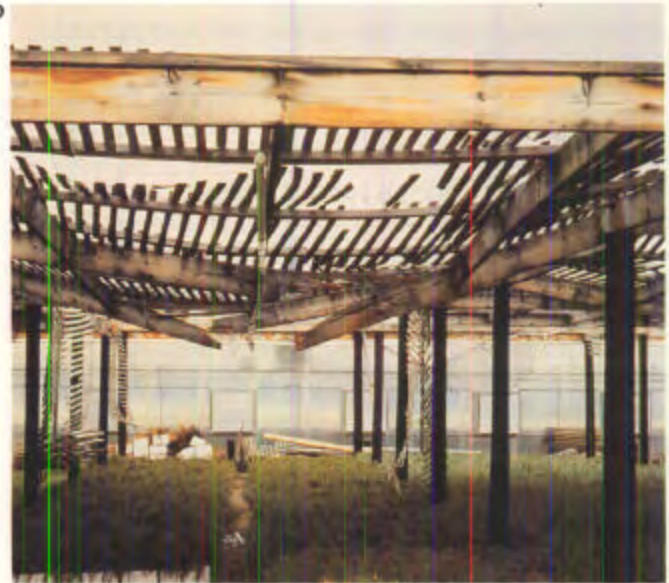
Figure 1.3.17 —Shadehouses are covered with lath (A) or shade cloth (B), which is now available in colors (C). Any type of growing structure must be designed to support structural loads, especially in snowy climates (D).
