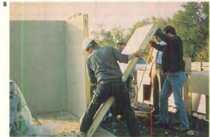
Figure 1.3.33 —Refrigerated storage buildings are commercially available in prefabricated modular units that can be easily installed either inside existing structures (A) or as separate buildings (B) (courtesy of Bally Engineered Structures).
