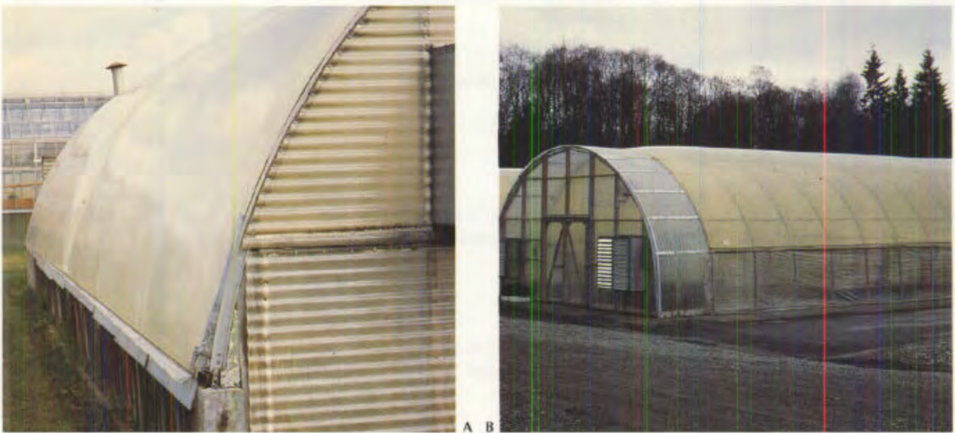
Figure 1.3.14 —Plastic (“poly”) sheeting is the most inexpensive way to cover (“glaze”) a propagation structure. Double-poly layers are air-inflated to provide a rigid covering (A), or a single layer can be installed over other coverings to increase the insulation value (B).
