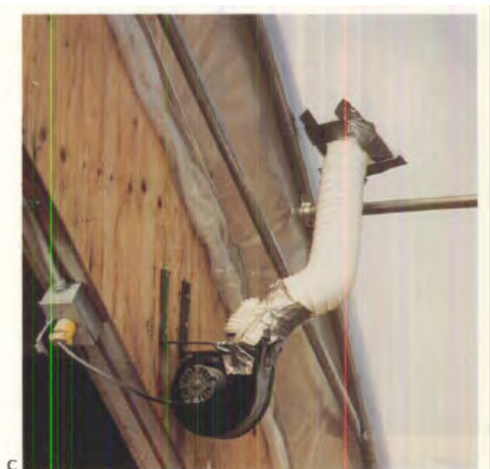
Figure 1.3.18 —Double layers of plastic sheeting can be attached to the framing with wooden furring strips (A) or specially designed fasteners (B), and a fan (C) maintains the positive air pressure to keep them inflated. (A, modified from Bartok 1993; B, from Hummert 1993.)
