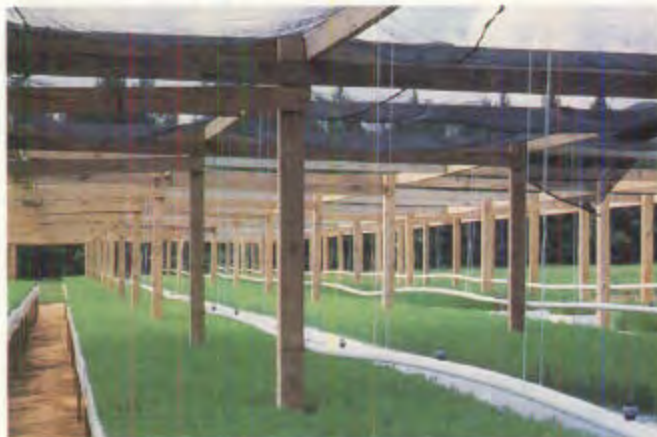
Figure 1.3.17 —Shadehouses are covered with lath (A) or shade cloth (B), which is now available in colors (C). Any type of growing structure must be designed to support structural loads, especially in snowy climates (D).
