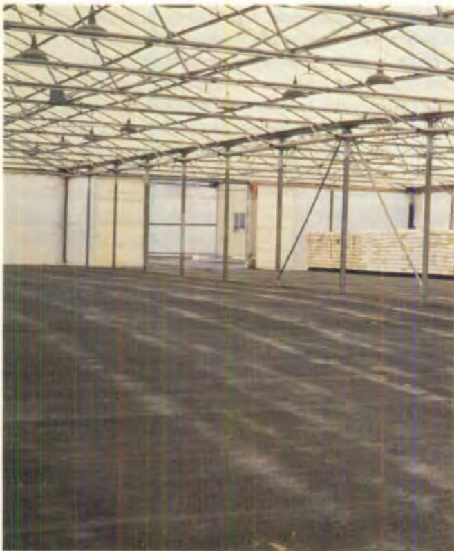
Figure 1.3.10 —Solid floors help keep the propagation environment clean and allow the use of handling equipment (A). Other structures feature traffic paths down the center aisle (B).
