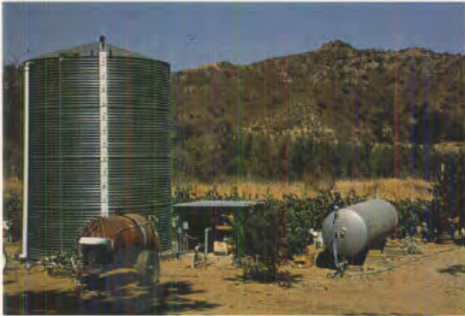
Figure 1.2.4 —if the flow from wells or streams is not enough to meet peak irrigation demand, it may be necessary to build water storage reservoirs or tanks.
