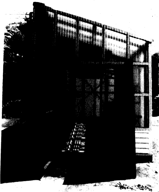
Figure 6-2.—Solar dryers are effective for drying seeds as well as lumber. Many designs exist; they are easy to construct and require little maintenance. The one shown here has fiberglass side and roof panels covering a treated wood frame.
