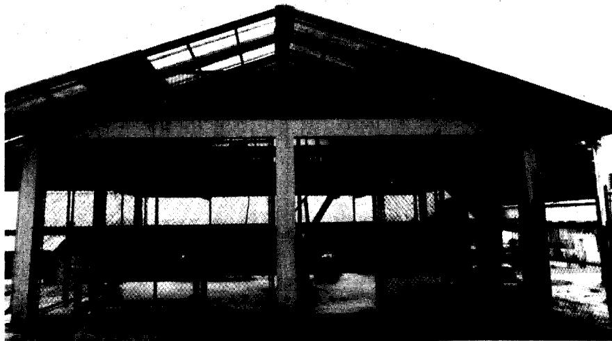
Figure 4-3.—Covered, open-sided nursery building that also doubles as lunchroom, seed extraction and drying area, and carpentry area for making small items such as shade frames for germination trays.
