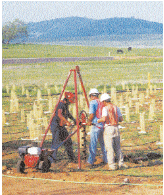
Figure 4. Installing 2 to 3.6 m (6 to 12 ft) cottonwood pole cuttings with a remotely powered Little Beaver™ auger, Yuba City, California.
