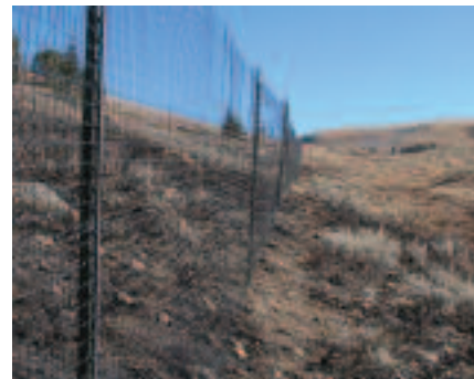
Figure 5. Plastic mesh fence, 7.5 ft tall (2.3 m), is supported by steel T-posts and high-tensile wire.
